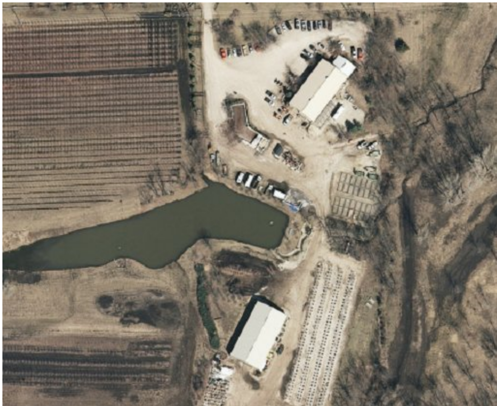
Aerial view of buildings on the subject property
